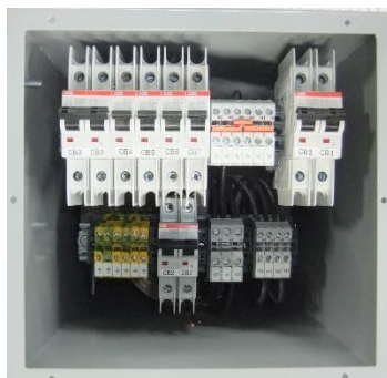
Pictured left: Top down view of 7.5kVA power center 480: 240/120 with (7) secondary MCBs. Pictured right: 800VAC metering cabinet (view door removed) with PTs and ION 8650 revenue grade meter.
